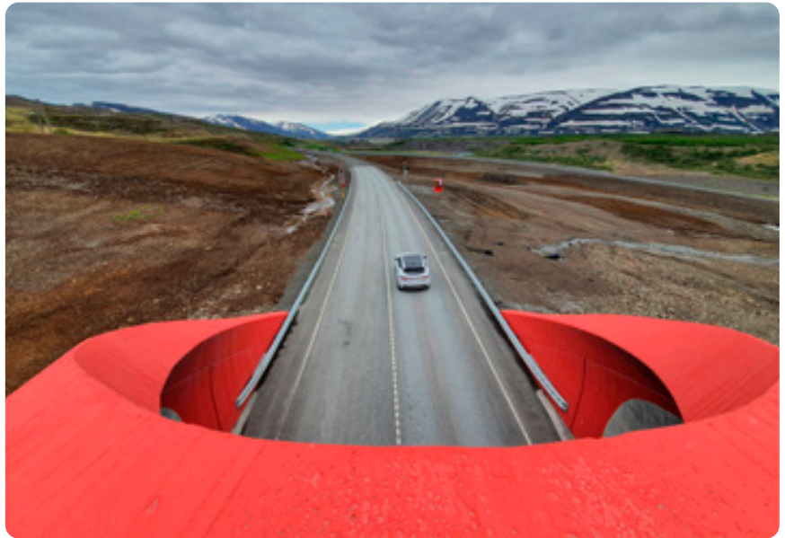
The tunnel bypasses the precipitous Víkurskarð Mountain Road, a hazard for drivers in bad weather
