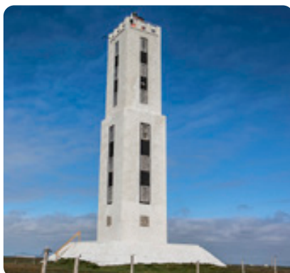
Built in 1938-1939, the Knarrarósvíti lighthouse was the first one in Iceland to be built out of reinforced concrete
